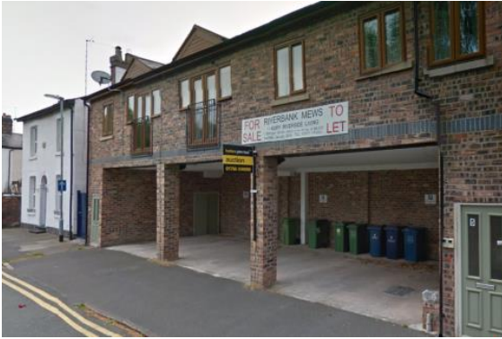
Figure XXX Undercroft parking which adds very little to character of the street scene
