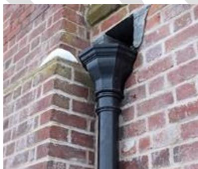
Figure XX An example of a decorative cast iron hopper these must be retained as they contribute to the character and appearance of the Conservation Area
