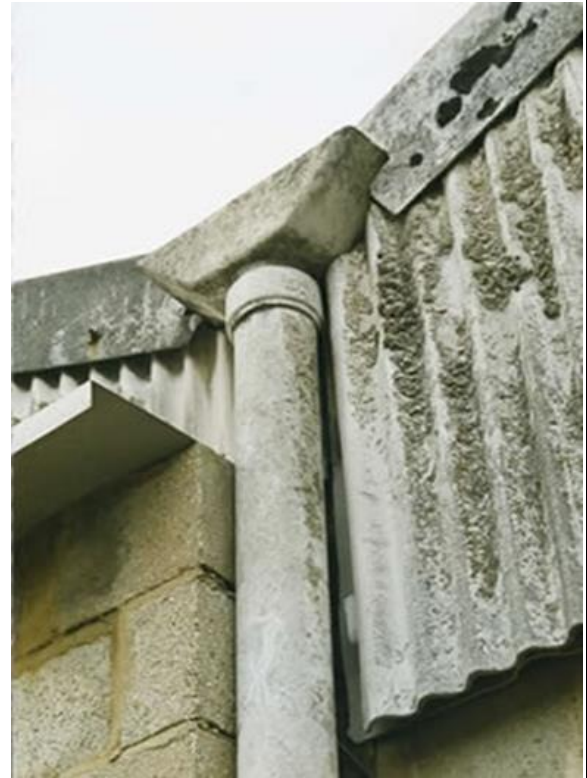
Asbestos cement downpipe, hopper and profile sheet
