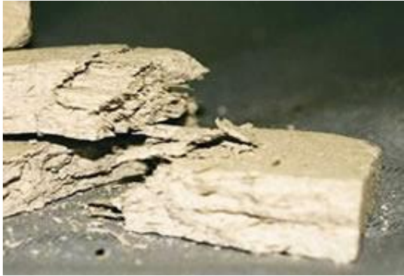
Pieces of Asbestos Insulating Board (AIB)
