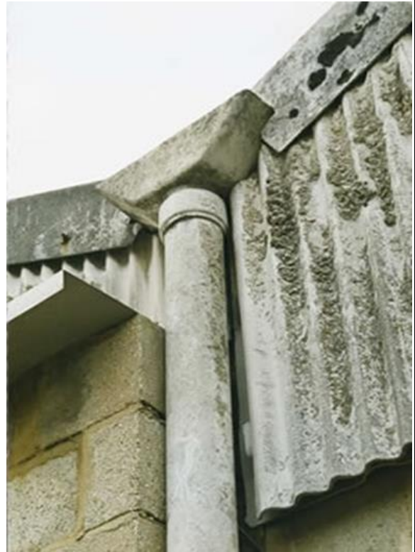
Asbestos cement downpipe, hopper and profile sheet
